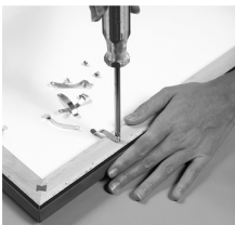
Secure with spring clips
